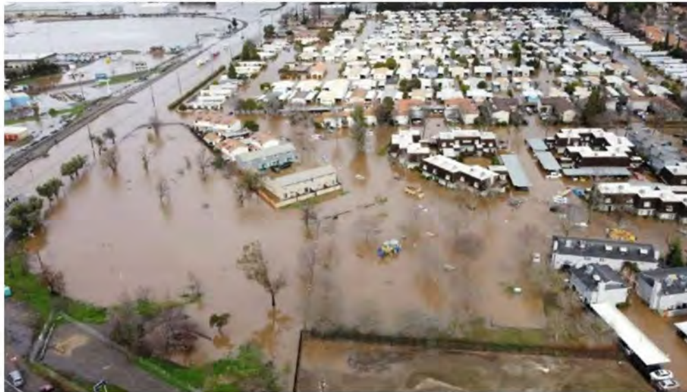
Water surrounds a neighborhood in western Merced after Bear Creek overflowed its banks in January 2023 storm. CITY OF MERCED
