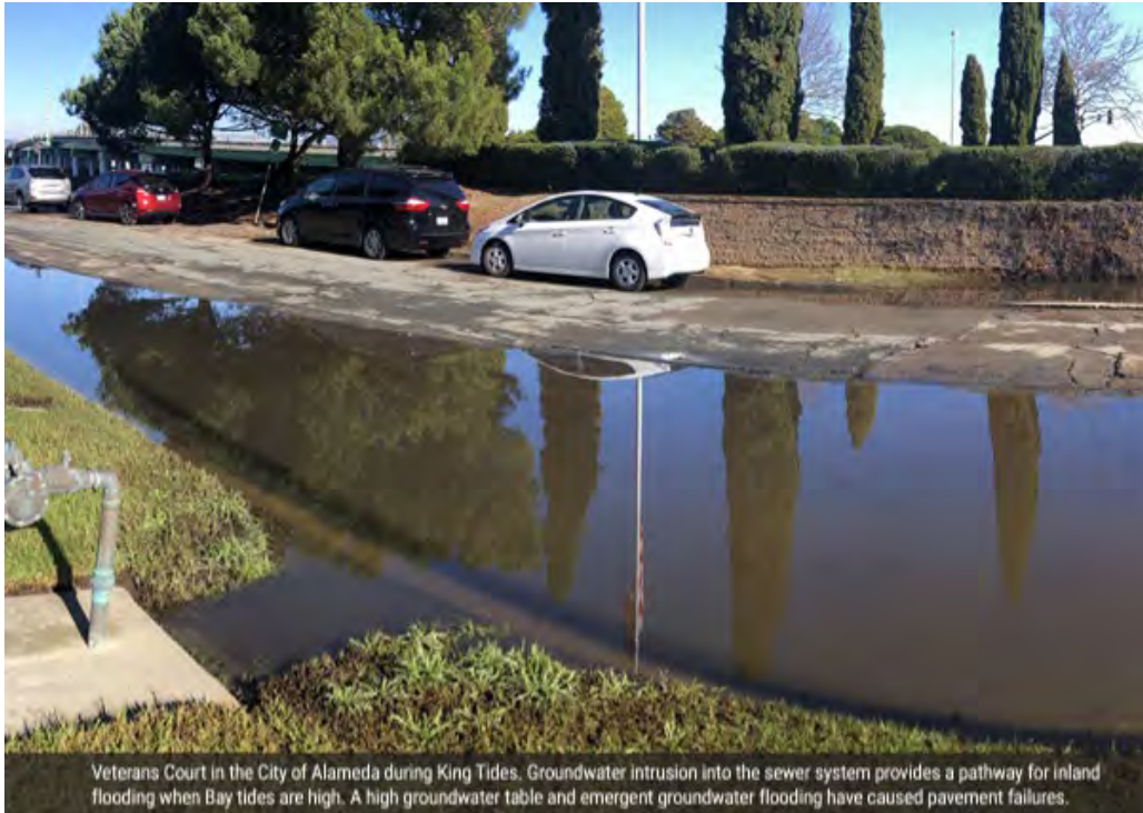
Photo of sunny day flooding from groundwater rise, from Shallow Groundwater Response to Sea-Level Rise by Pathways Climate Institute and SFEI, 2022.
