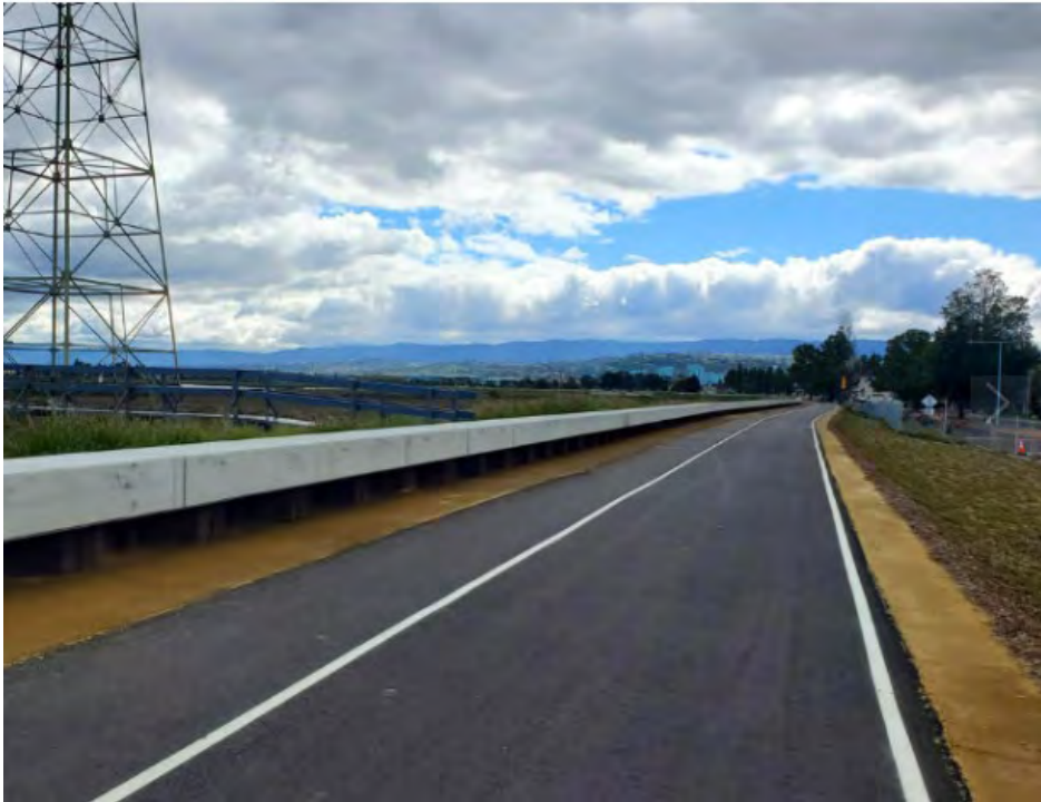
A sheetpile wall on a levee in Foster City: Fostercitylevee.org
