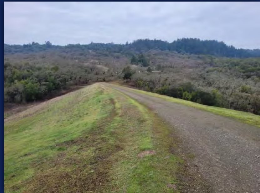
Dam Embankment - Facing South
