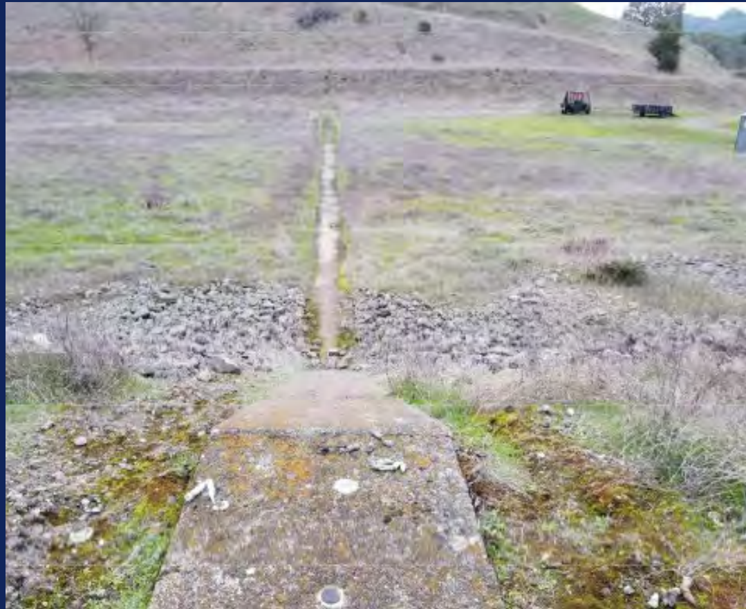
Auxiliary Spillway Structure
