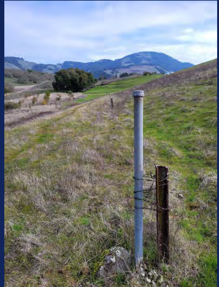
Downstream Stability Berm (Facing North)
